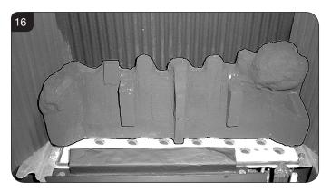
812 Place the front coal centrally in the channel at the front of the tray. The relationship between the front coal and the flame baffle is shown, Diagram 17.
