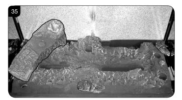
9.20 Place Log B on top of Log D. There is a hole on the underside of Log B which fits over the raised stud on Log D to secure in place. The right hand side of the log rests in the groove in the burner, see Diagram 36.
