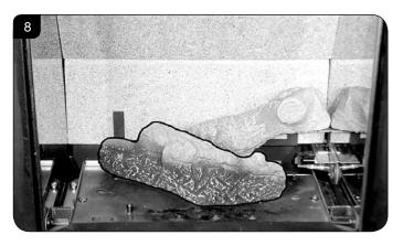
7.4 Place Log E onto the stud and behind the tag on the left hand side of the burner tray.Rest against Log B, see Diagram 9.
