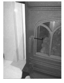
2. Slide the door handle over the hex nut ensuring that the handle is in the downwards position. Using the Allen key and grub screw (supplied) secure the handle in position.
